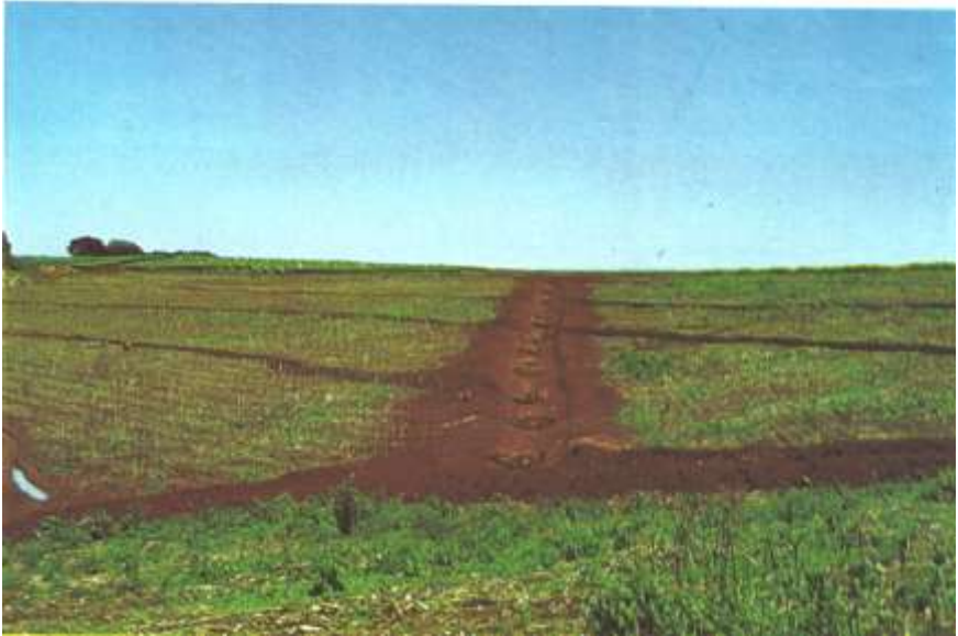
Plate 2: Main drain prepared before grassing but with the field staked ready for planting
