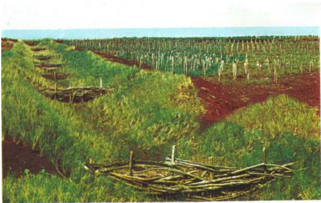
Plate 2 Main drain grassed with Eragrostis curvula to protect it from erosion.
